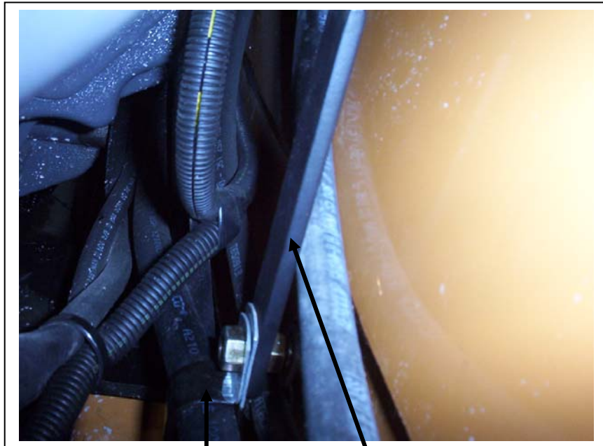
Heater hose bracket in the new location
